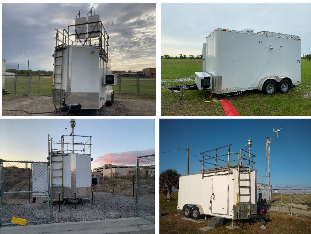
Figure caption: Clockwise from top left: (BC) 2 trailers at Aldine, West Liberty, Galveston, and El Paso. Both Galveston and El Paso had Digital samplers installed inside with inlets through the roof, while Aldine and West Liberty had URG samplers which were installed outside on the walkable roof.
