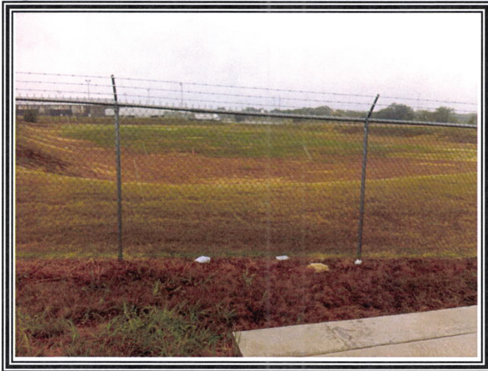
11. View southwest from near the northern limit of the north wastewater line. Detention pond feature S-2 is in the background.
