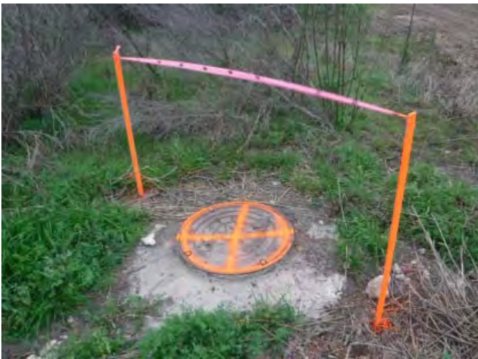
View of Potential Recharge Feature # S-63.
