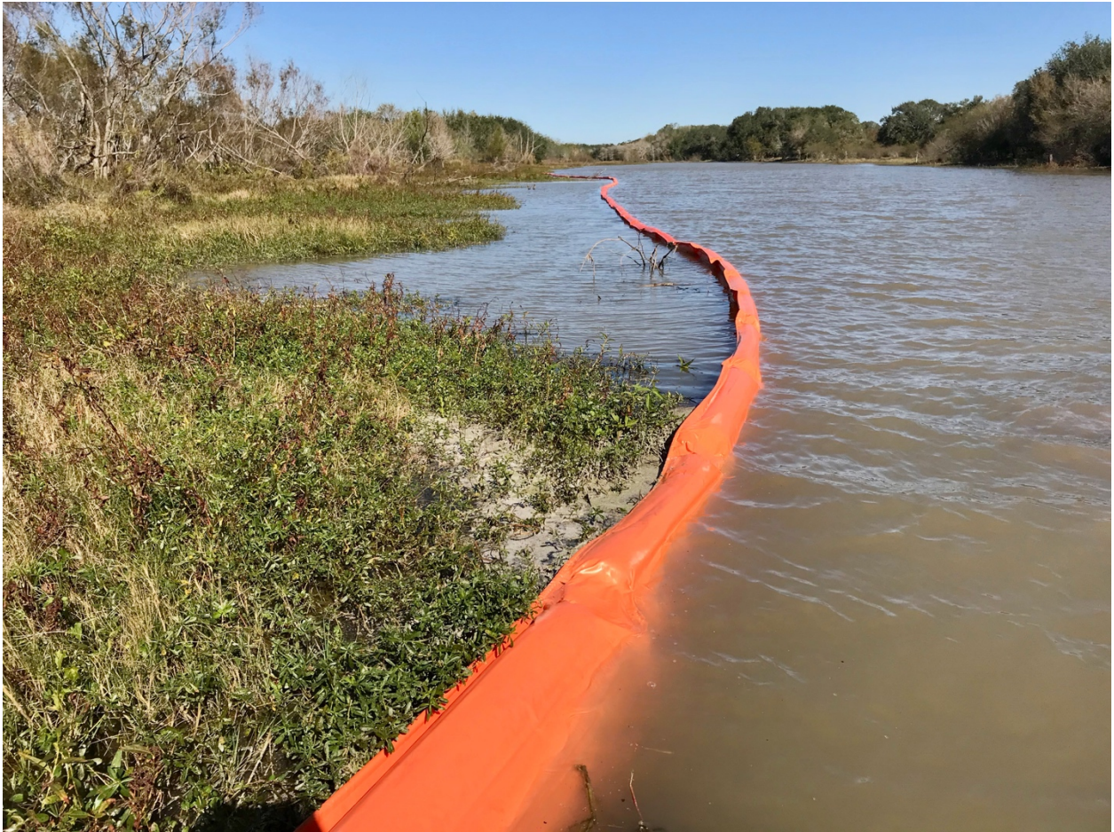
Figure 8. Film of plastic powder captured by boom positioned near Outfall 009.
