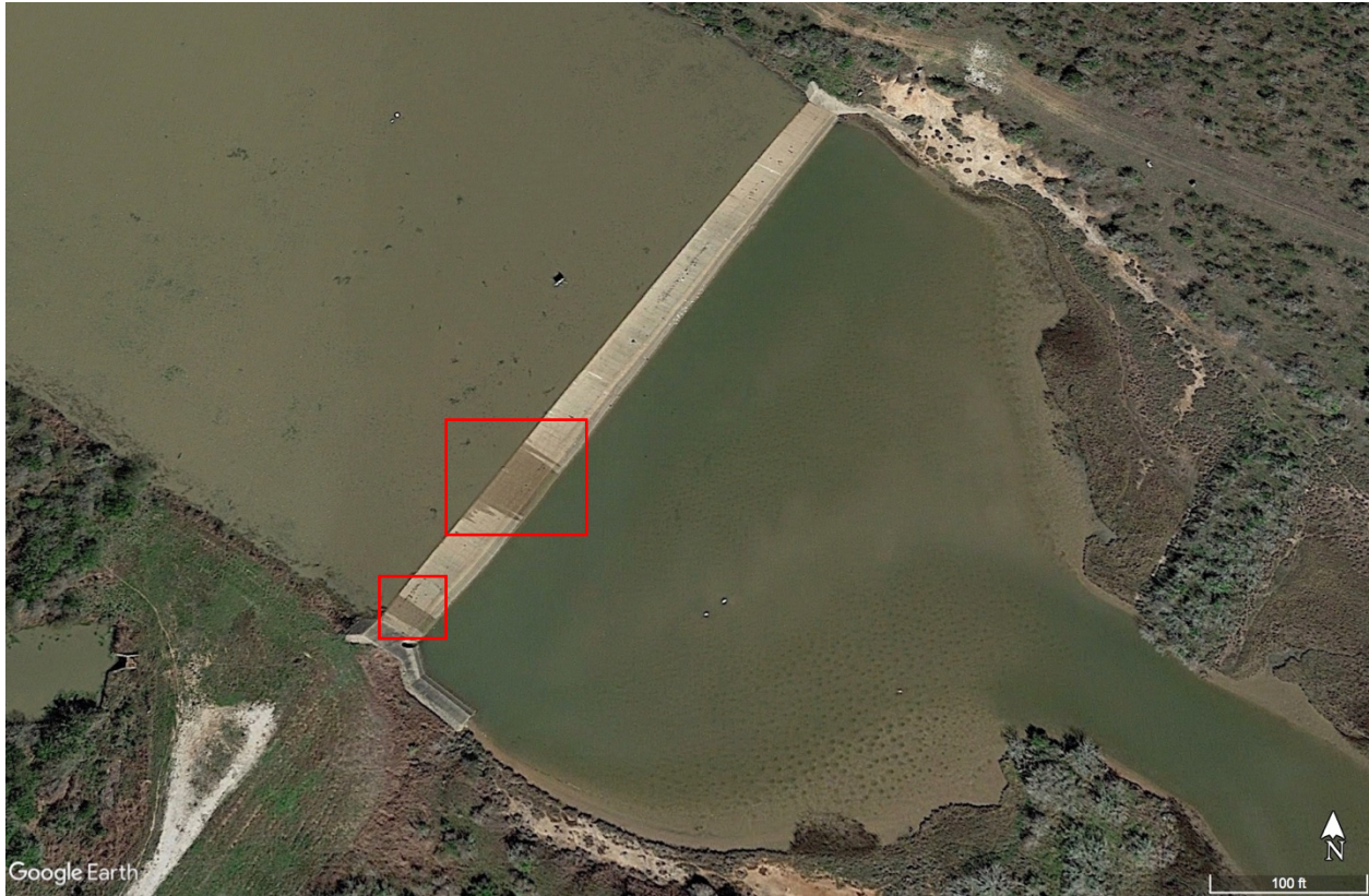
Figure 29. Image of Cox Creek spillway dam on Google Earth from February 2003. Most of the dam is dry, with only 2 small areas (red boxes) allowing water to flow into the downstream marsh. This indicates that the water does not always flow from Cox Creek in to the marsh.
