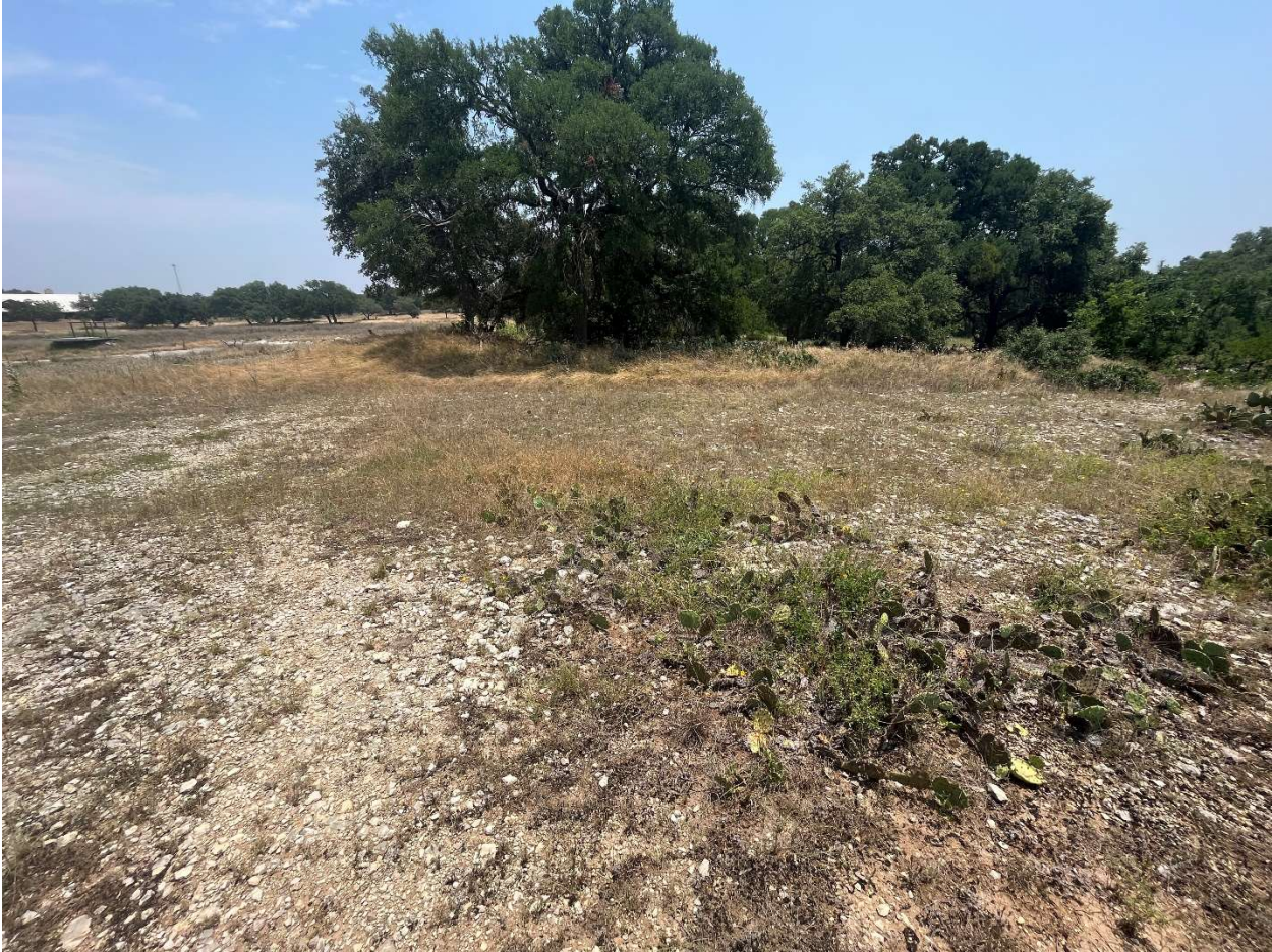
Photo 18 – Looking Southeast from approximately 170 feet from the Southwest corner of the dam
