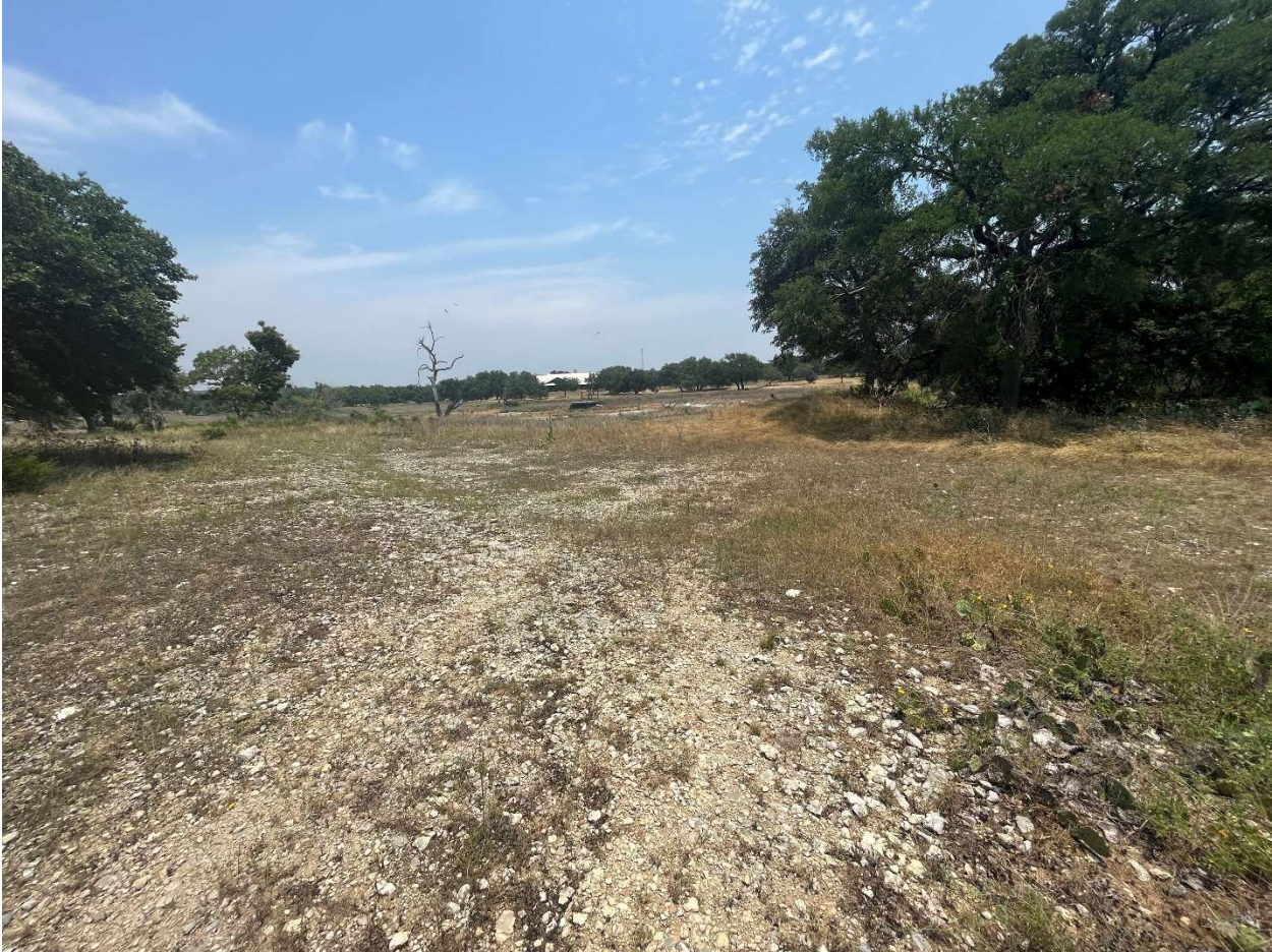
Photo 17 – Looking Northeast from approximately 170 feet from the Southwest corner of the dam
