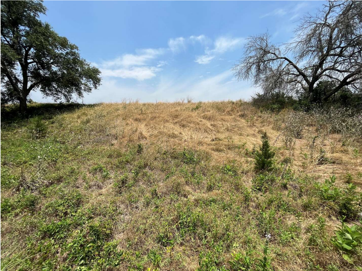
Photo 14 – Looking North from approximately 80 feet south of the dam
