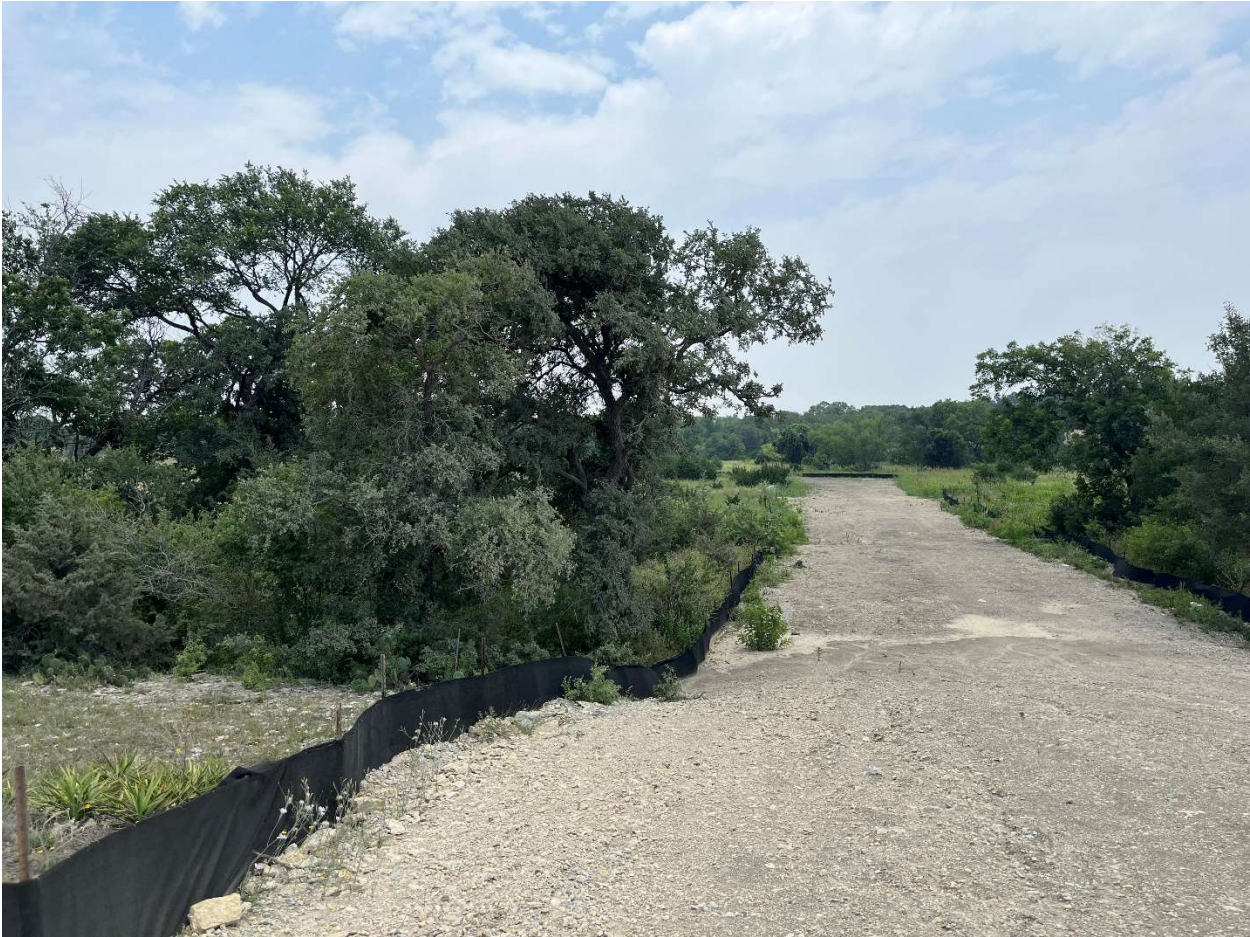
Photo 13 – Looking Northeast from approximately 100 feet south of the pond
