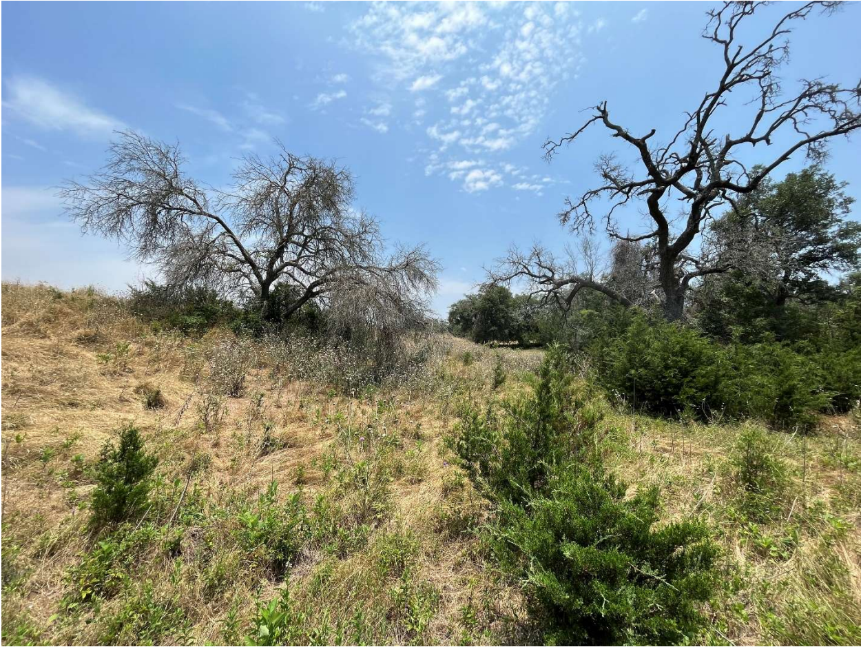
Photo 15 – Looking East from approximately 80 feet south of the dam
