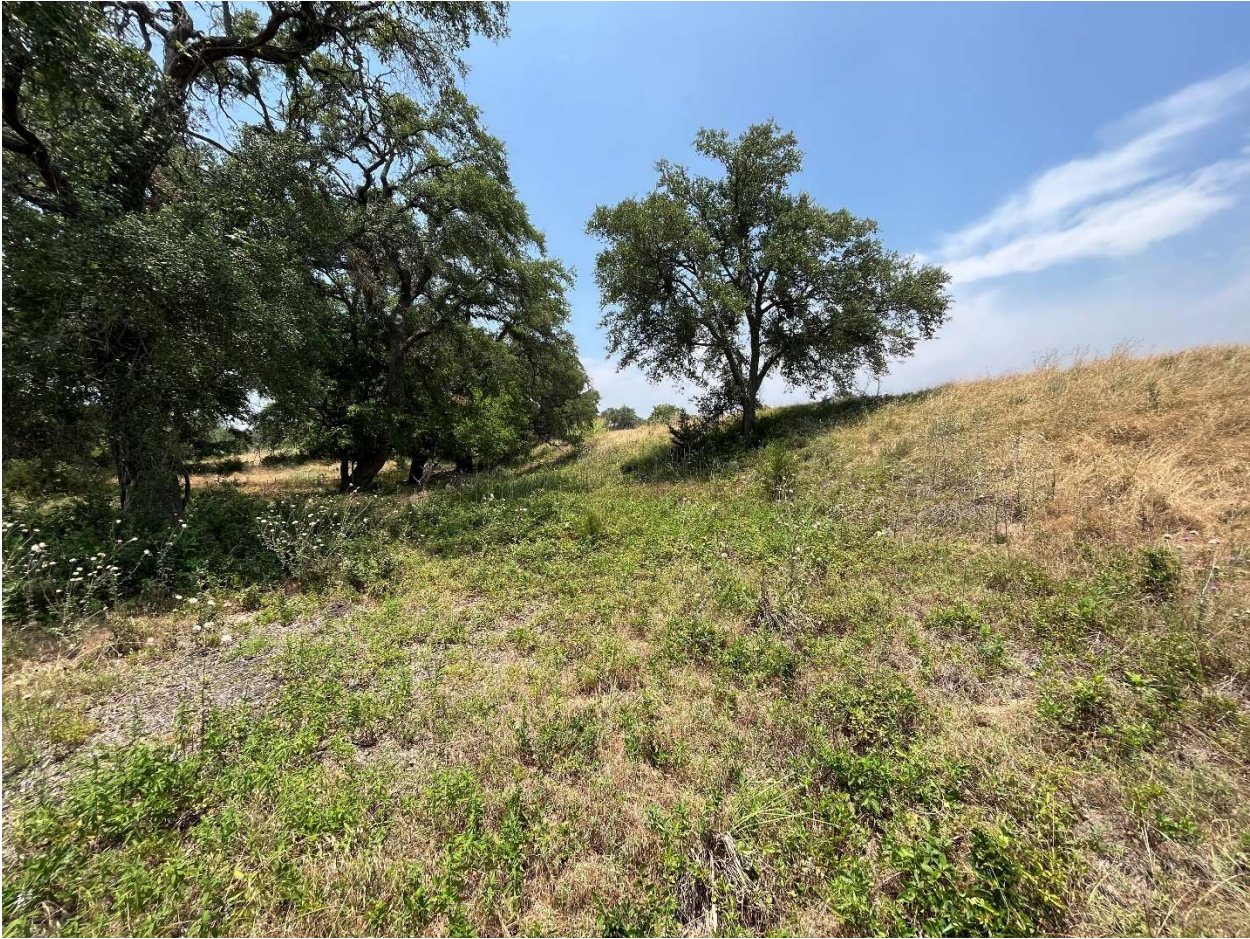
Photo 13 – Looking West from approximately 80 feet south of the dam
