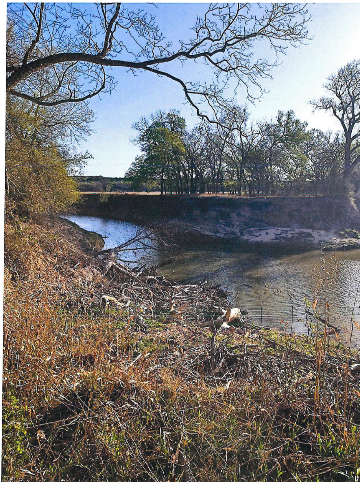
Photo 3: (Reach B-B') Downstream Limit B' Looking Upstream
